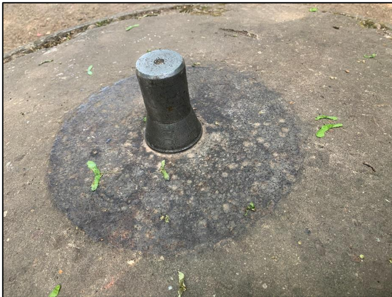
Figure 5: Steel Pintle atop spigot mortar platform
